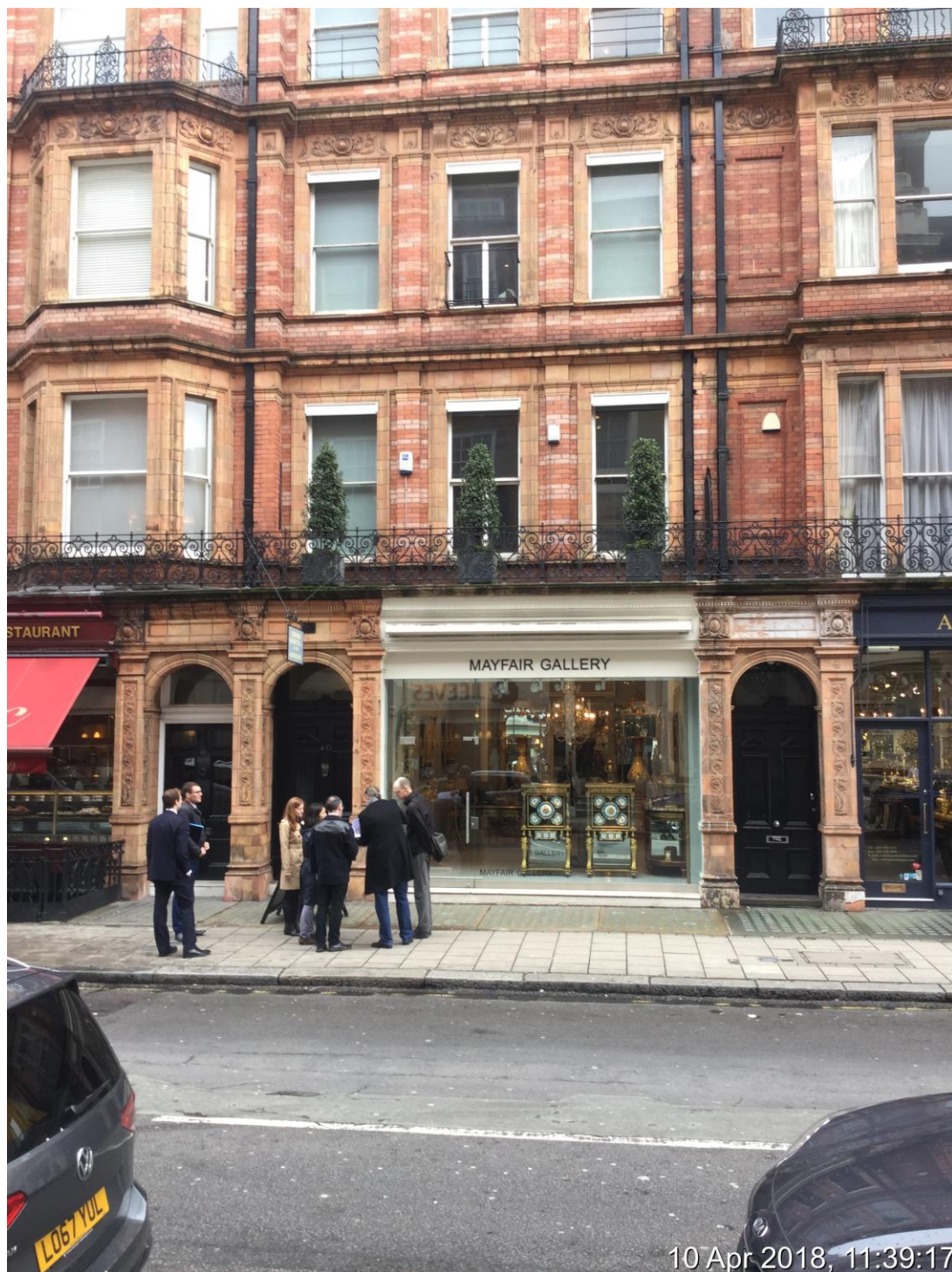
South Audley Street Frontage
